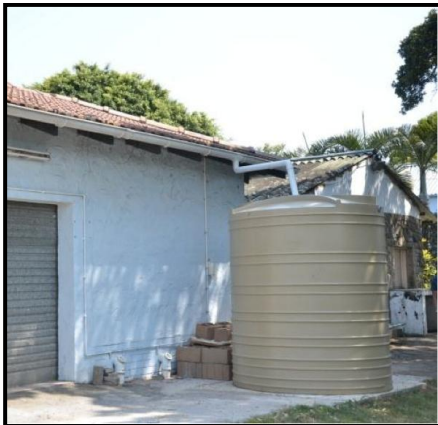
The new 'Jojo' water tank donated by Action Udobo
